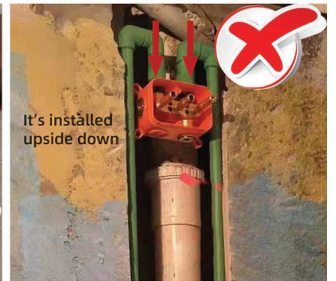
The installation of concealed plastic box in wrong way
